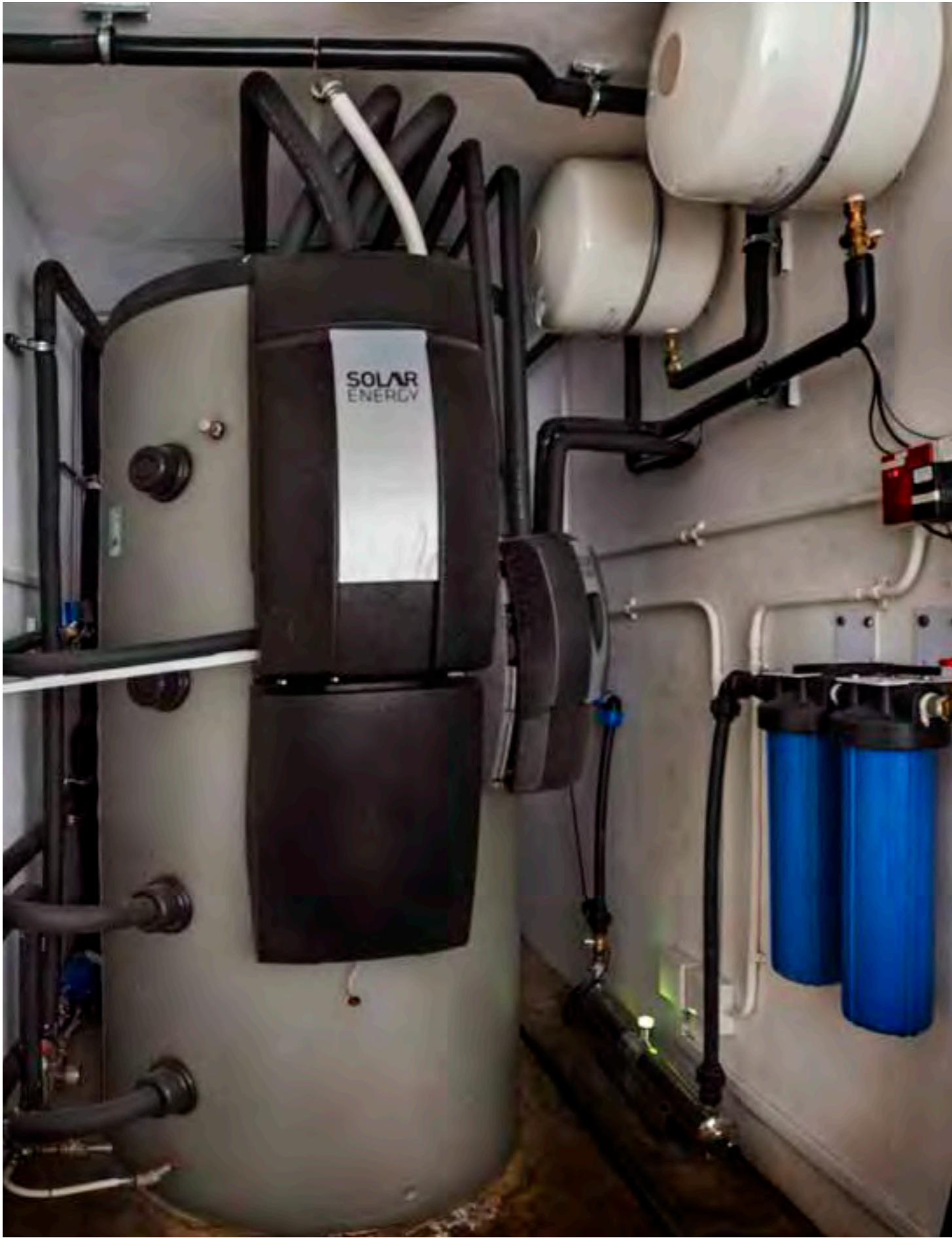
IMAGE 21: 100 LITRE STORAGE TANK BATTERY AND WATER TREATMENT EQUIPMENT
