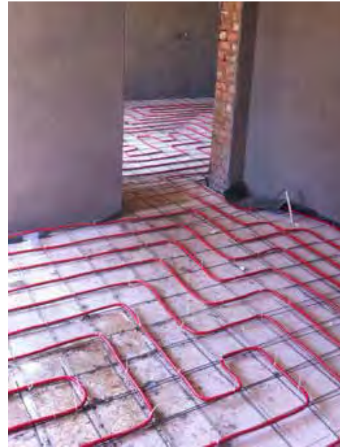
IMAGE 23: UNDERFLOOR HEATING PIPES LAYOUT
