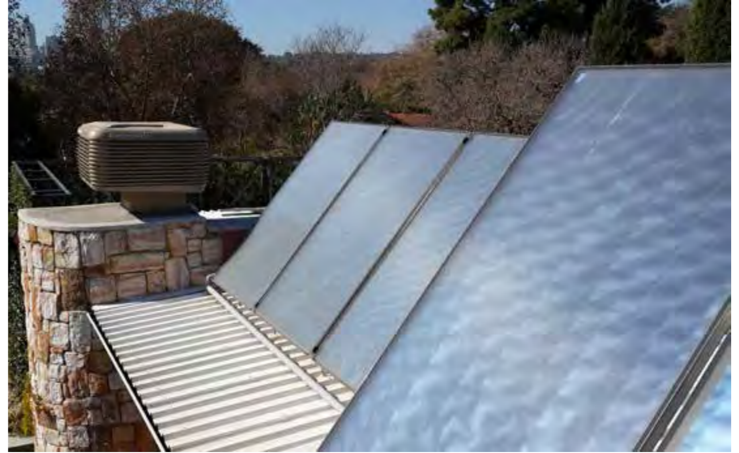
IMAGE 22: SOLAR WATER HEATING PANELS
