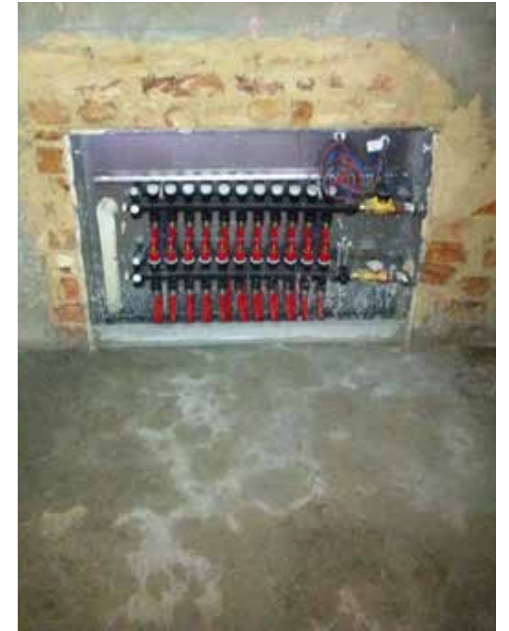
IMAGE 24: UNDERFLOOR HEATING PIPE MANIFOLD
