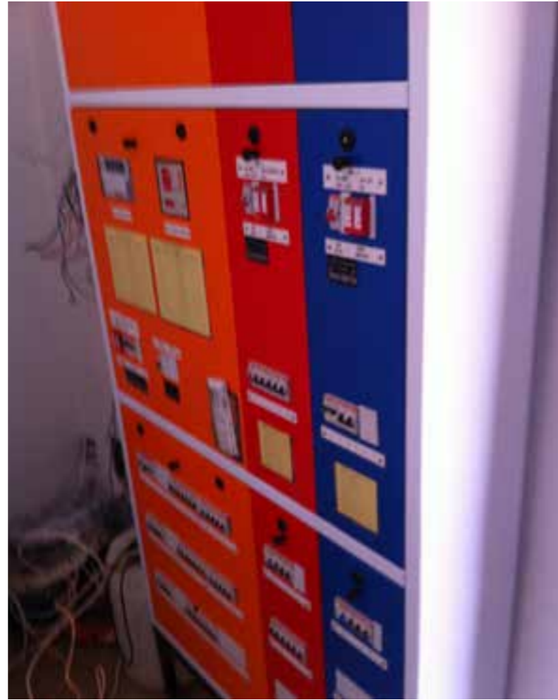
IMAGE 15: COMPLEX DISTRIBUTION BOARD
