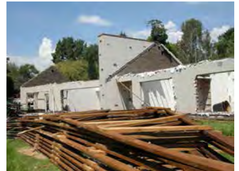
IMAGE 03: SOFT STRIPPING STRUCTURAL MATERIAL
