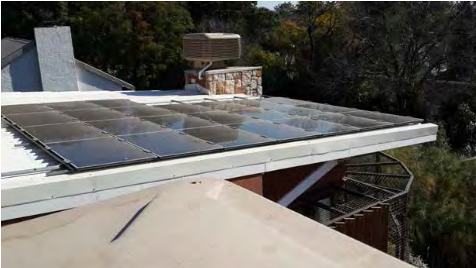
IMAGE 16: PHOTO VOLTAIC PANEL ARRAY
